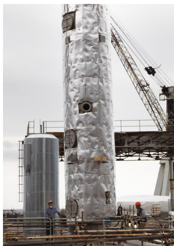
The ECO-EGC™ OPEN LOOP system, uses only seawater to neutralize the SO 2 contained in the exhaust gas.
